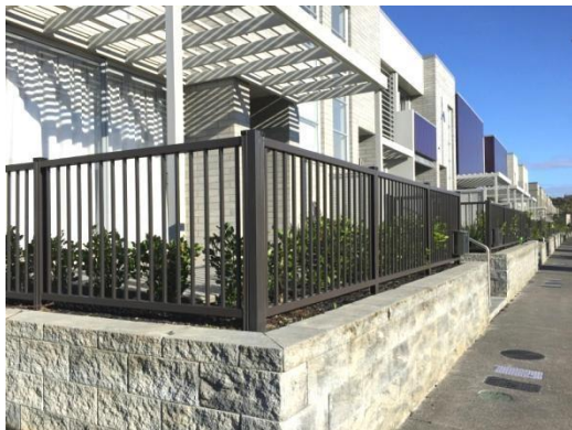
Figure 2: Moduline safety fence installed in concrete pile footings behind a retaining wall
